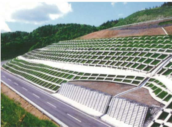
Slope stabilization
