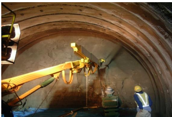
TBM Tunnel Linings
