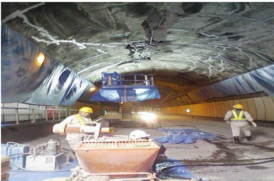
Rock support in tunnels and mines
