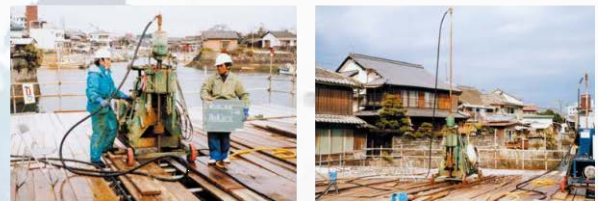
Application to Various Types of Soil Improvement
