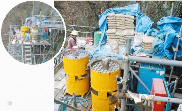
Application to Slope Face (Rock Collapse Prevention)
