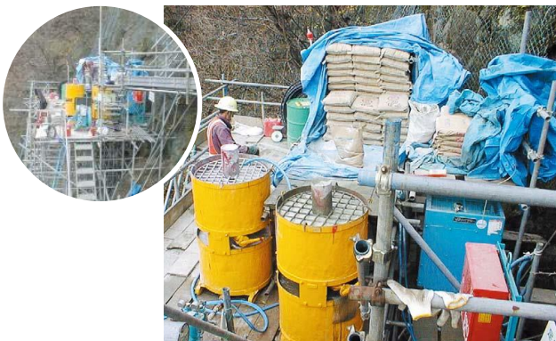
Application to Slope Face (Rock Collapse Prevention)
