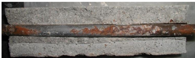
Plain concrete : Corrosion present
